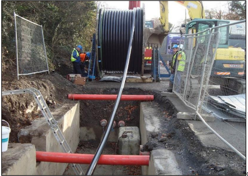
Figure 5-5: Photo of cable pulling procedure.
