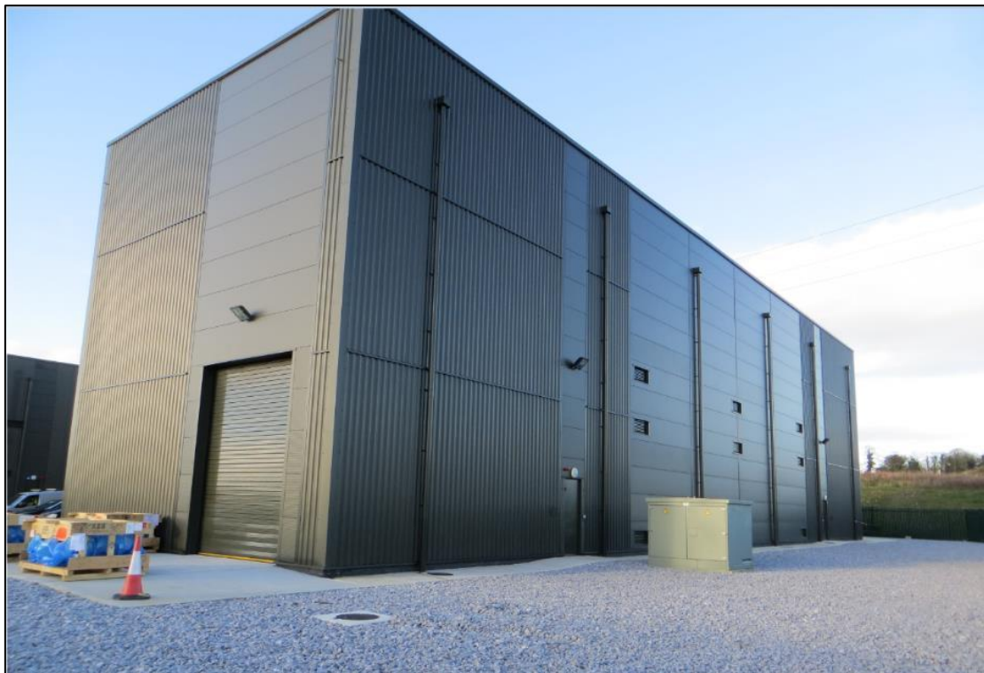
Figure 5-6: Photo of 220 kV GIS Substation Building.
