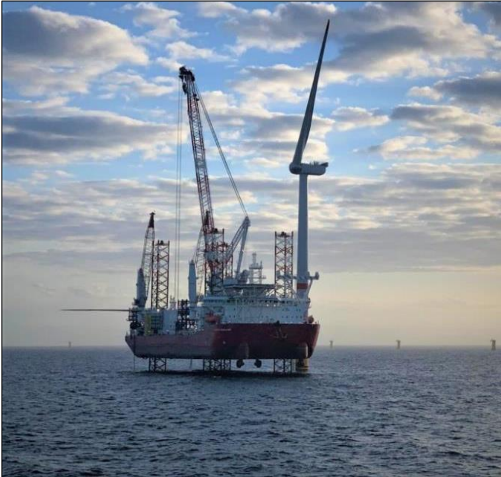
Figure 5-3: Installation vessel installing wind turbine blades.
